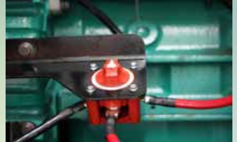
Battery Isolator Switch
